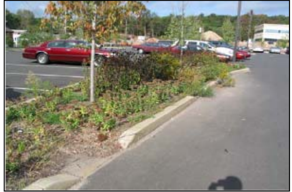
Bio-retention Area at Staples Parking Lot Branford, Connecticut
