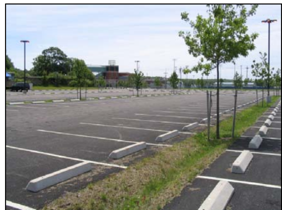
Porous Asphalt Parking Lot University of Rhode Island, Kingston
